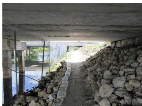
I-75 Alligator Alley bridge after panther ledge installed. Photo courtesy of FDOT.
